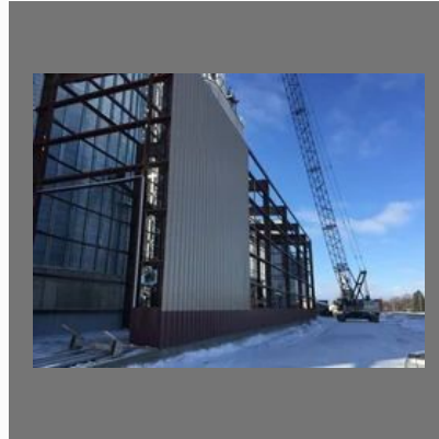
Pre Engineered Metal Buildings Construction Service
